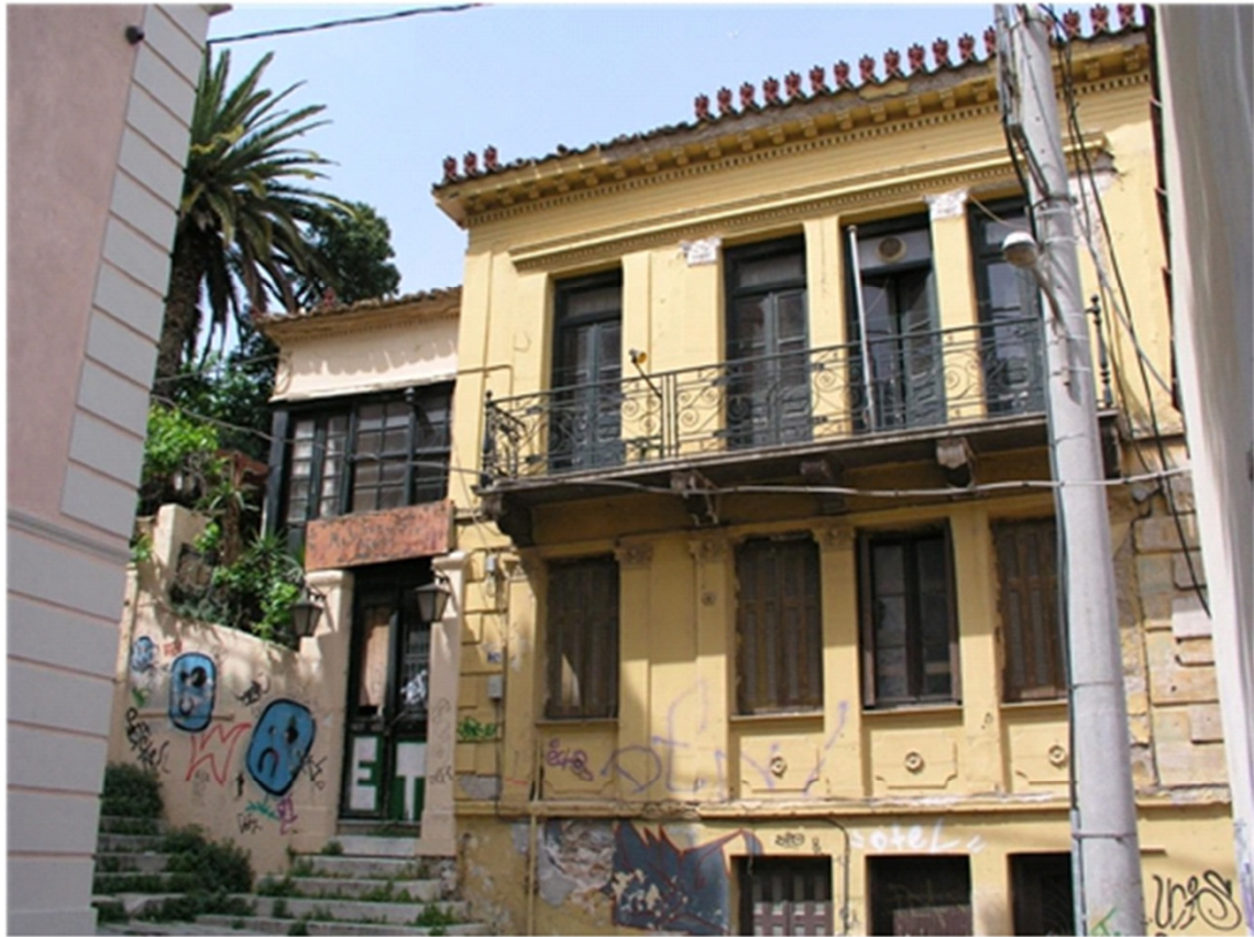
Athens. Another example of a house hiding a traditional layout behind the symmetrical and inflexible neoclassical façade.
