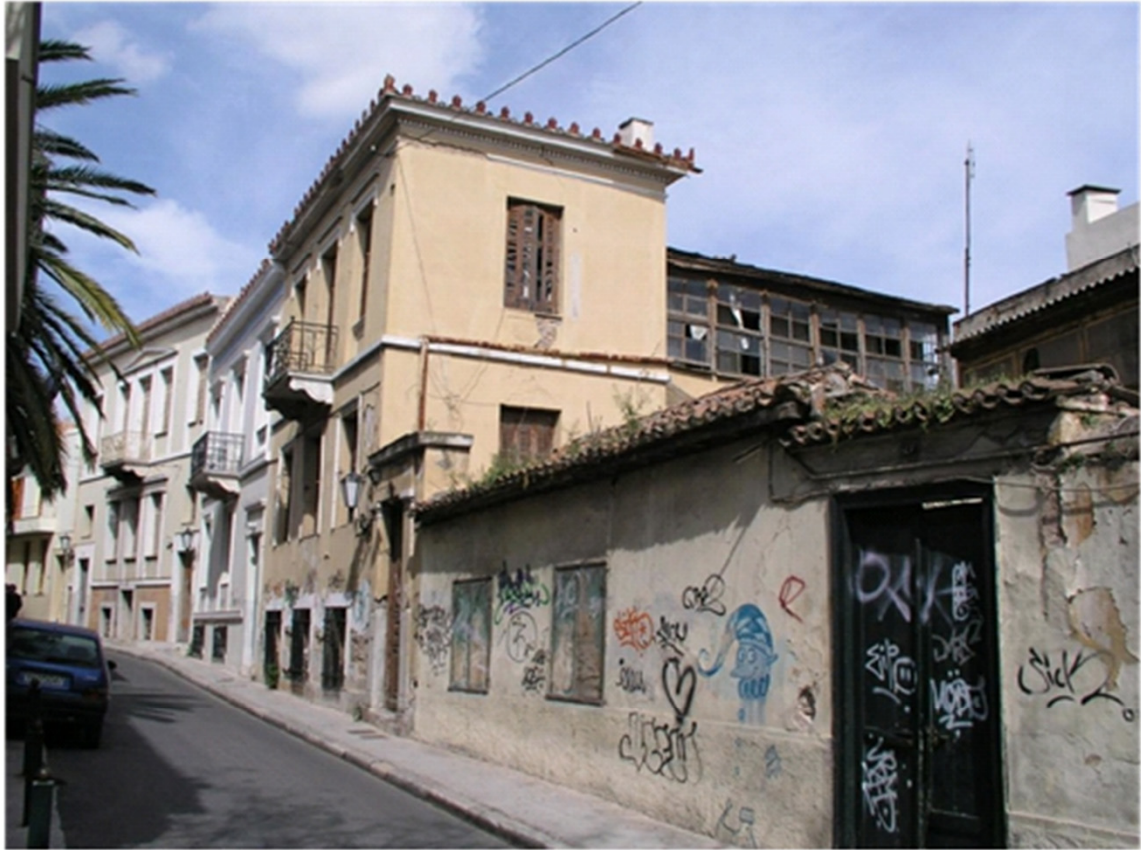
Athens. A house hiding a traditional layout behind the symmetrical and inflexible neoclassical façade.
