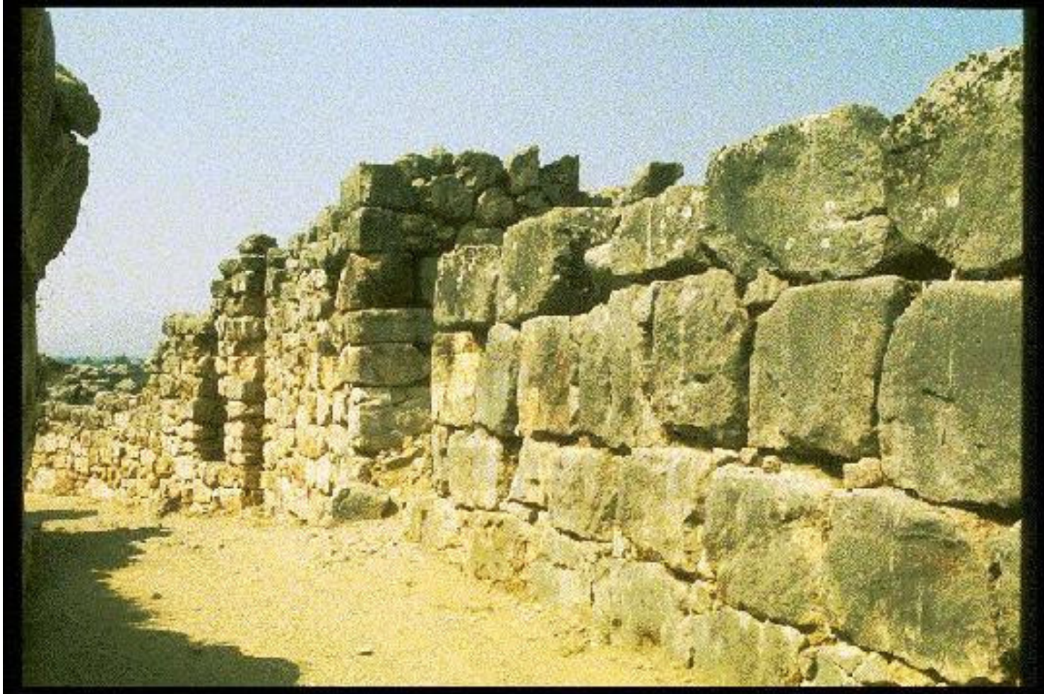
Cyclopean Walls at Tiryns
