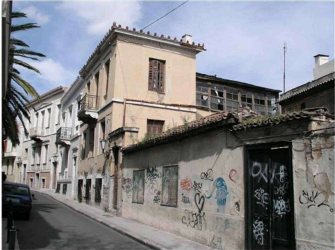
Athens. A house hiding a traditional layout behind the symmetrical and inflexible neoclassical façade.
