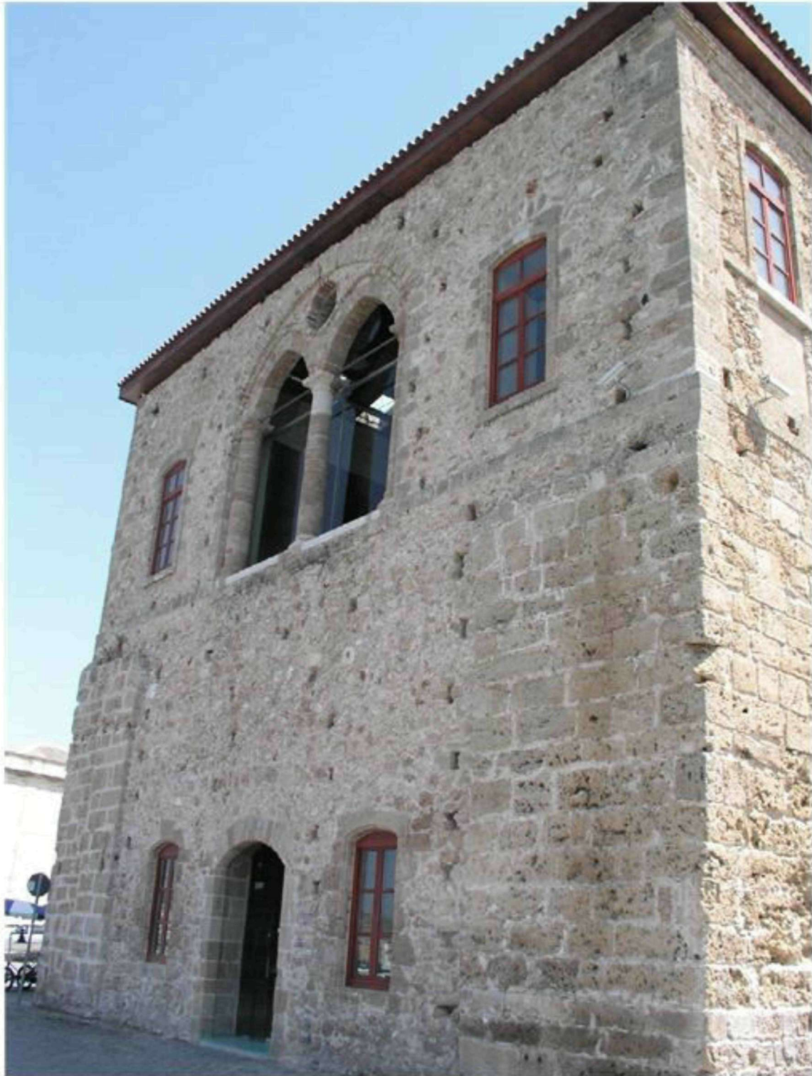
Chania, island of Crete. Vaulted loggia in a 15 th century Venitian arsenal. Its today use as a cultural centre led to the addition of glass panes.
