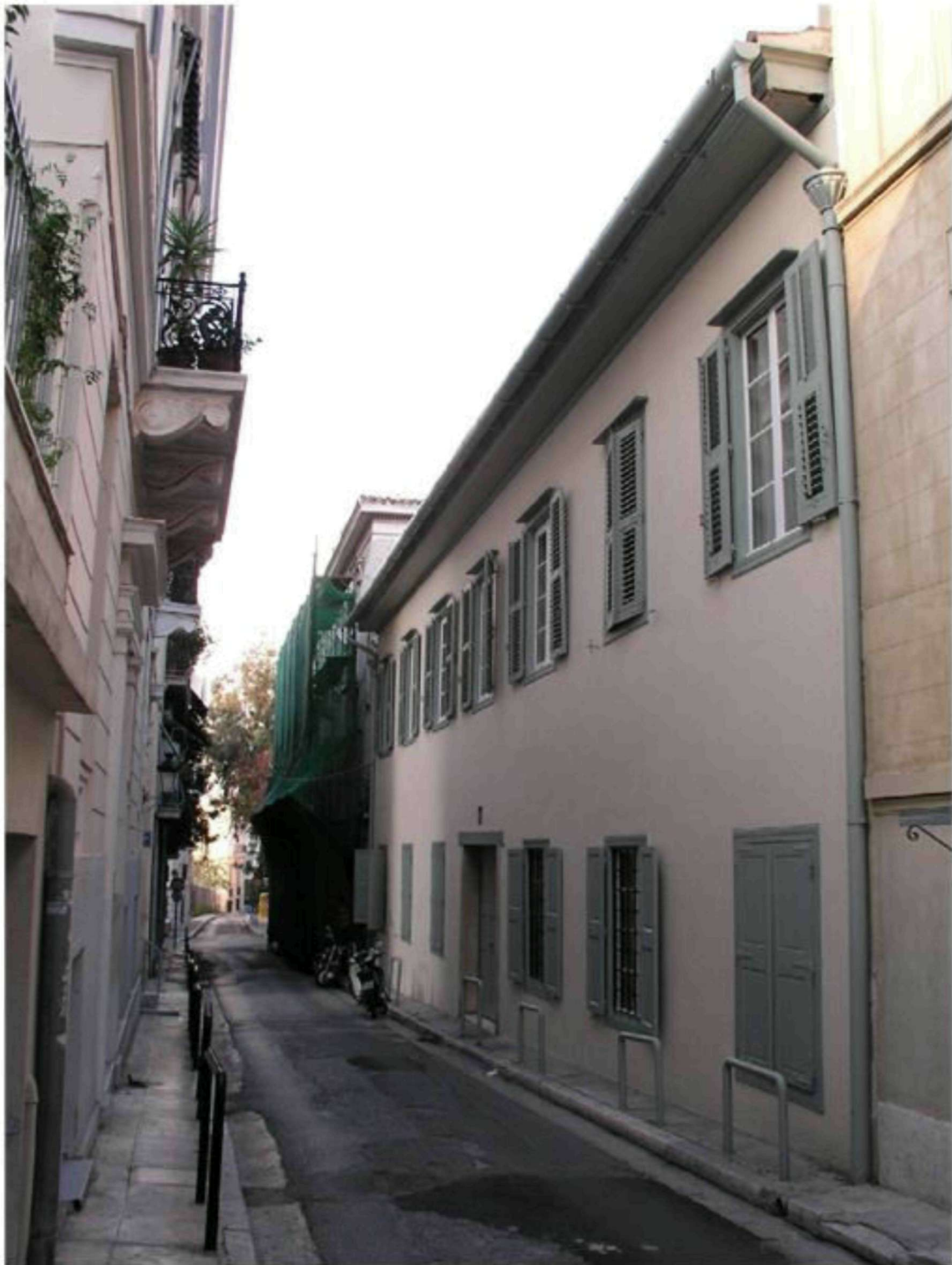
Athens. An example of a house hiding completely its traditional and highly bioclimatic layout behind its symmetrical and rigid façade. It is the house with the balcony closed with glass panes presented previously.
