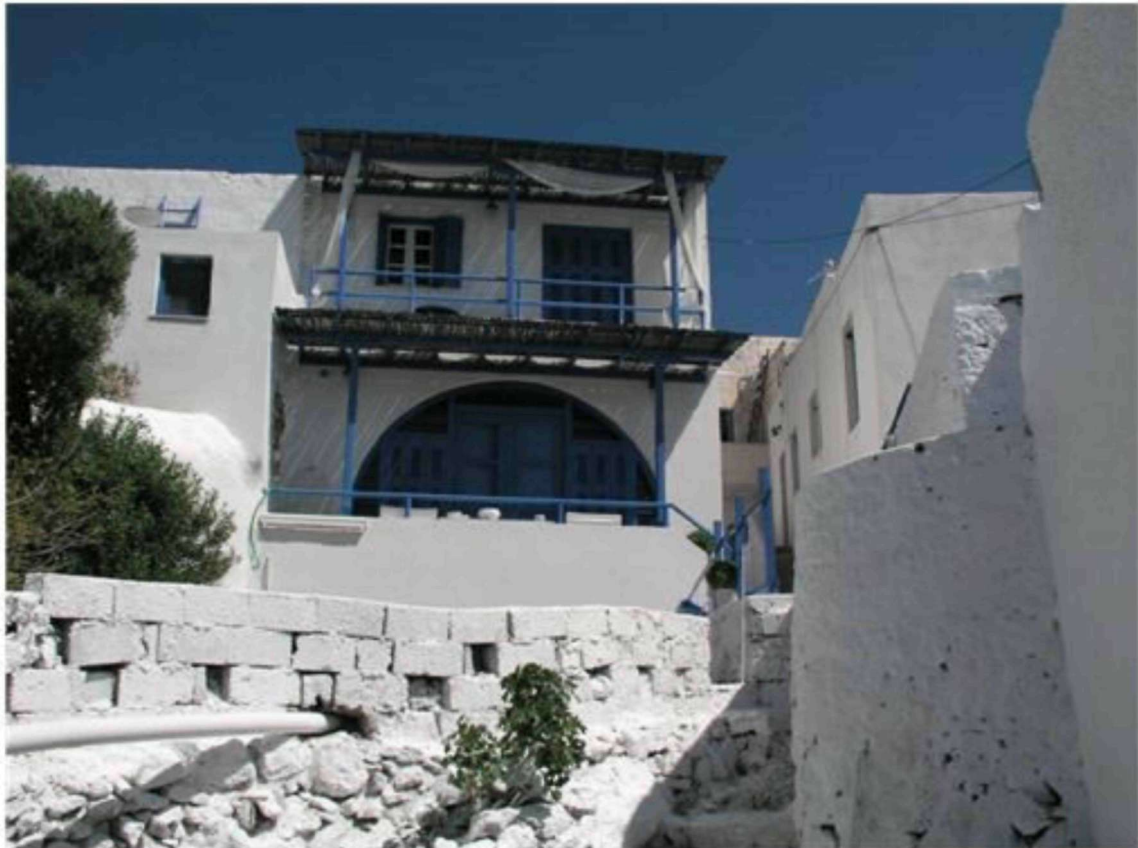
Island of Milos. A modern house adopting traditional forms (due to legislation imposing it). Vaulted loggia and cane shelter.
